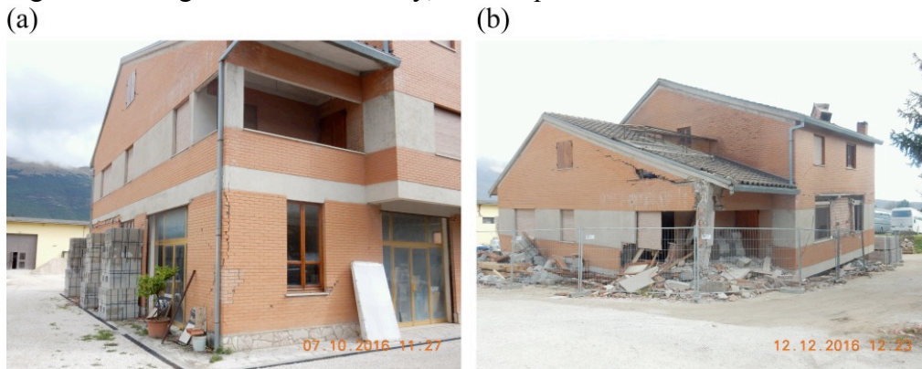
Figure 9. Reinforced concrete residential building (a) after the first earthquake and (b) after the entire sequence.
