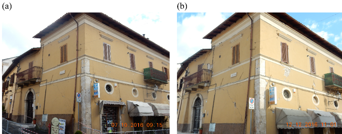
Figure 7. Masonry residential building (a) after the first earthquake and (c) after the entire sequence.
