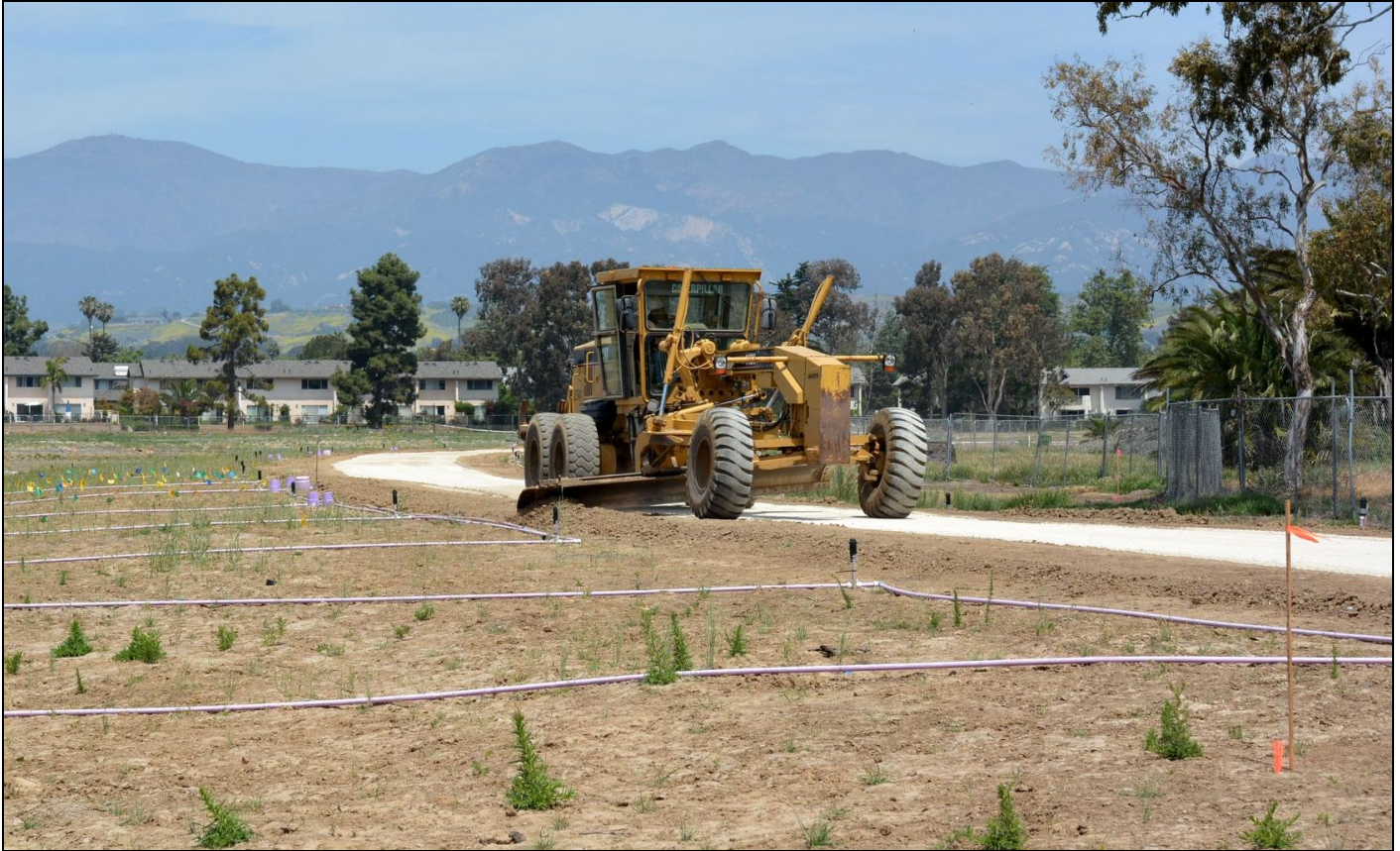
Contractors grading and smoothing the trail along the east side of NCOS.
