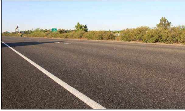
Figure 5.2: Orland Control, June 2011 (24 months). Note ruts in wheelpath.
