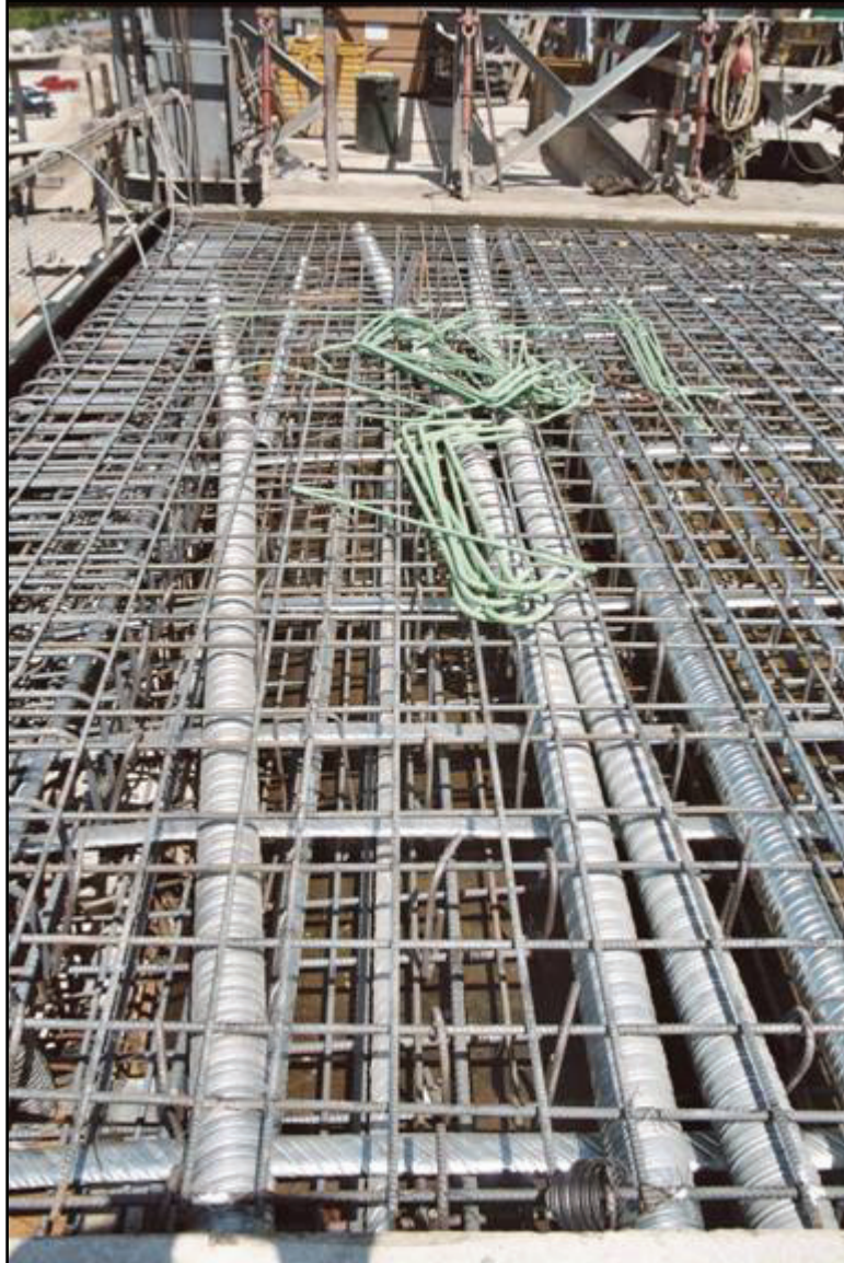
Figure A-13-36 SFOBB Deck Reinforcement and PT
