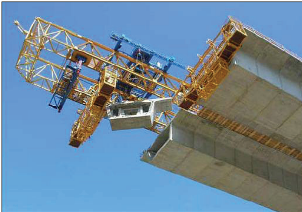
Figure A-13-48 Otay River Bridge - Segment Installation (Courtesy of Parsons)
