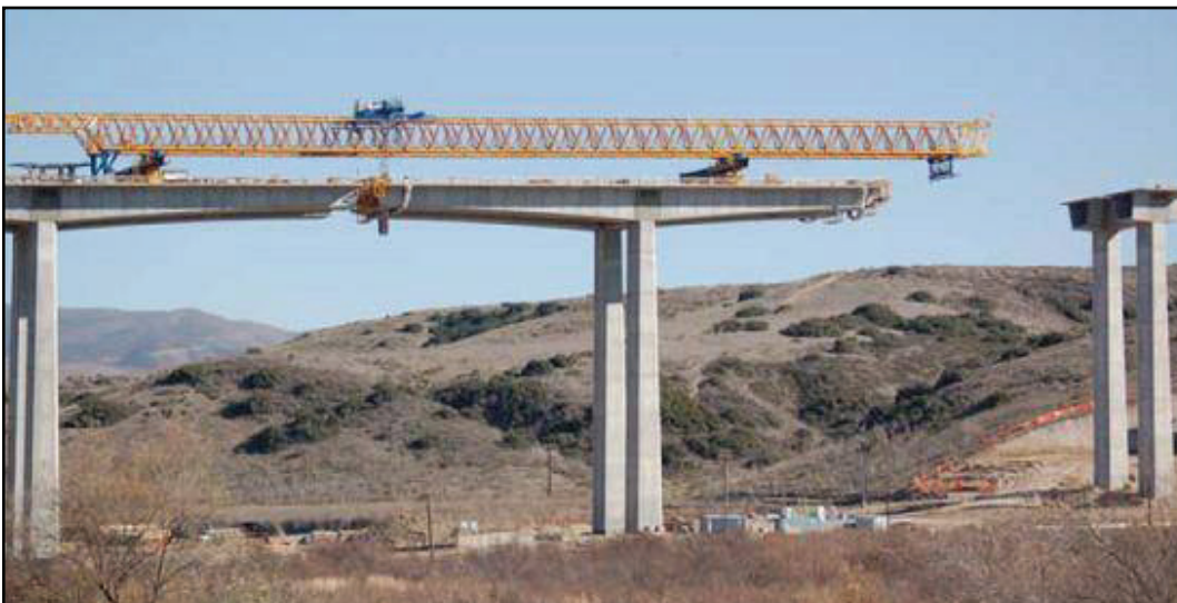
Figure A-13-52 Otay River Bridge (Courtesy of International Bridge Technologies)
