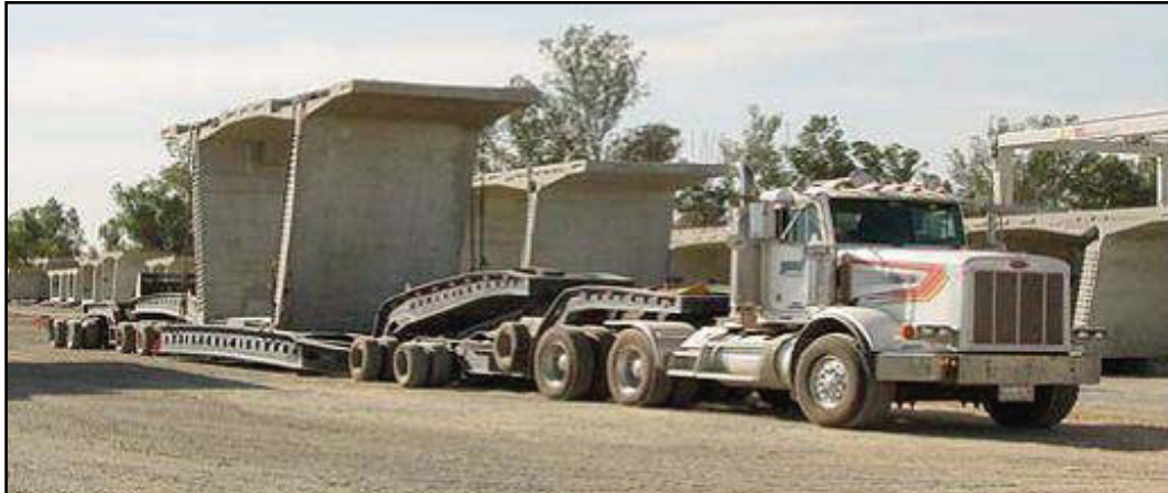
Figure A-13-45 Otay River Bridge - Transport of Segment (Courtesy of International Bridge Technologies)
