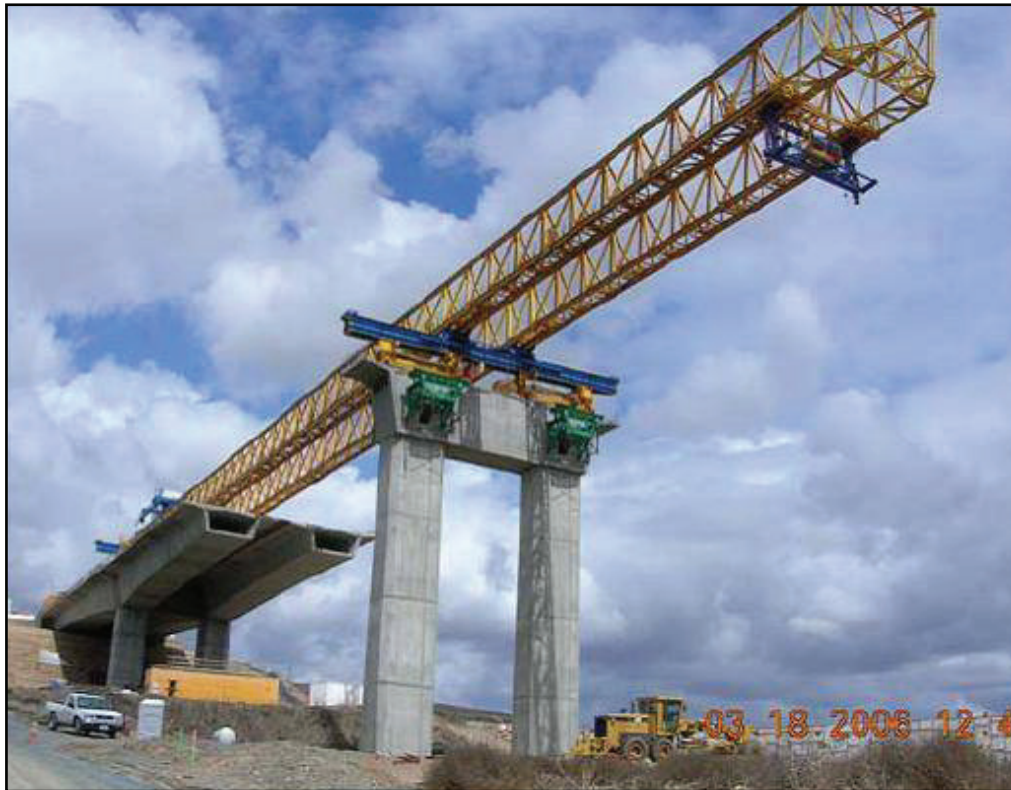
Figure A-13-47 Otay River Bridge – Overhead Erection Gantry (Courtesy of Parsons)
