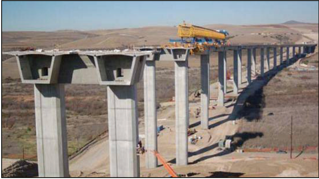
Figure A-13-53 Otay River Bridge (Courtesy of International Bridge Technologies)
