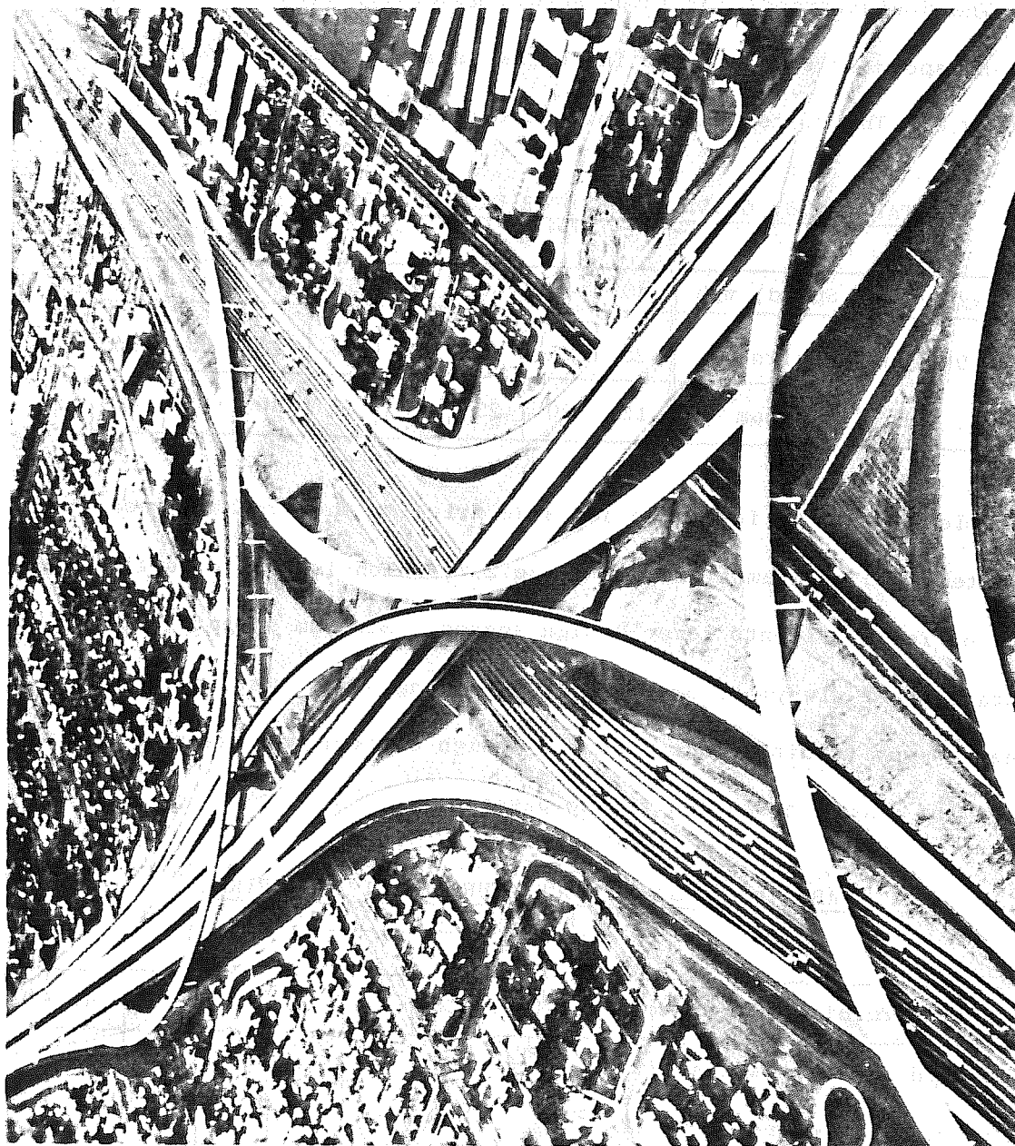
Fig. 2.7 Interchange Between San Diego and Santa Monica Freeways in Los Angeles (Courtesy of California Highway Department)
