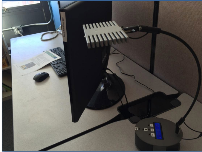
Figure 19: Initial Readings-At-Desk Controller Prototype Installed in FLEXLAB®
