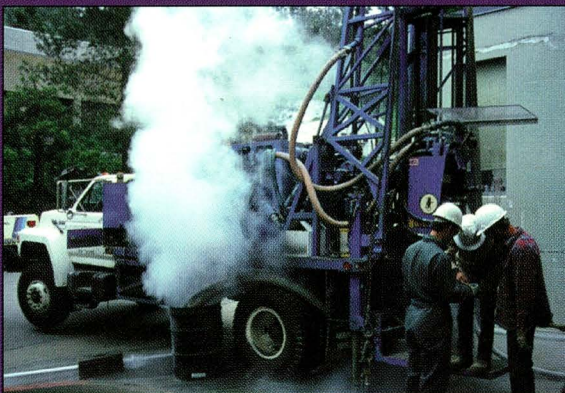
Berkeley Lab has developed cryogenic drilling, a technique used for drilling environmental monitoring and remediation wells in unstable soils and rock by freezing the borehole wall with nitrogen. (Contact: Sally Benson)
