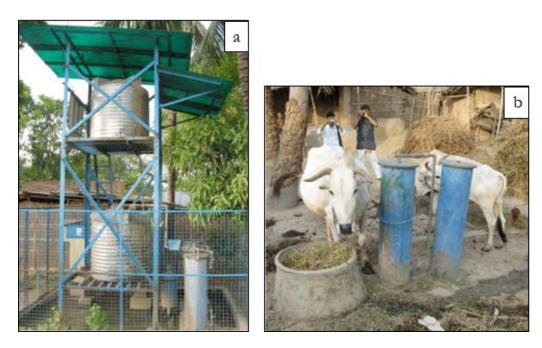
**Fig. 5.1** Photographs of arsenic treatment devices in Murshidabad District of West Bengal, India. Panel a), Working arsenic filter, (typical for 5% of installed units at 1-year after installation). And, Panel b), Defunct arsenic treatment unit, (typical of 95% of units at 1-year after installation)
