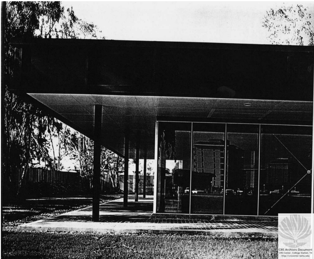
2.7. Prototype school on Stanford's Campus. Taken from SCSD: The Project and the Schools: a report from Educational Facilities Laboratories , 25. Courtesy of CRS Center, Texas A&M University, College Station, Texas.
