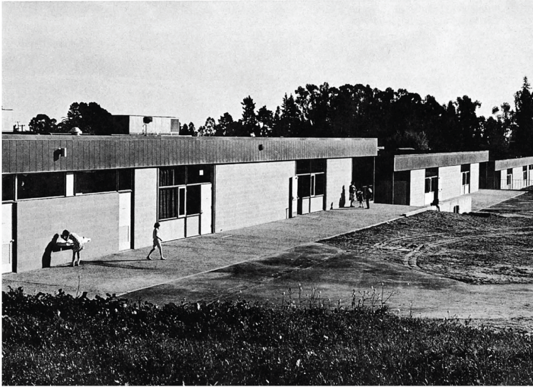
3.4. DeLaveaga School. Taken from "School Construction Systems Development Program," Arts and Architecture , April 1967.
