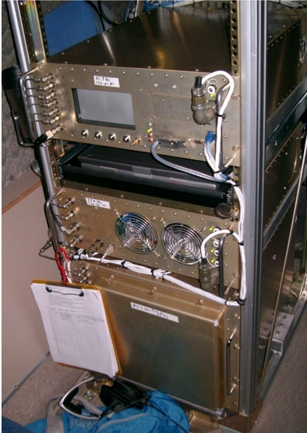
Figure 2.11. The operator side of the AO2 instrument seen from the aisle of the GV. The cylinder box sits at the bottom of the rack, with the pump box and instrument boxes above it. The system is run by an internal computer, accessed remotely from the data display laptop shown retracted in the laptop tray, though some interaction is also possible through the front panel of the instrument box.
