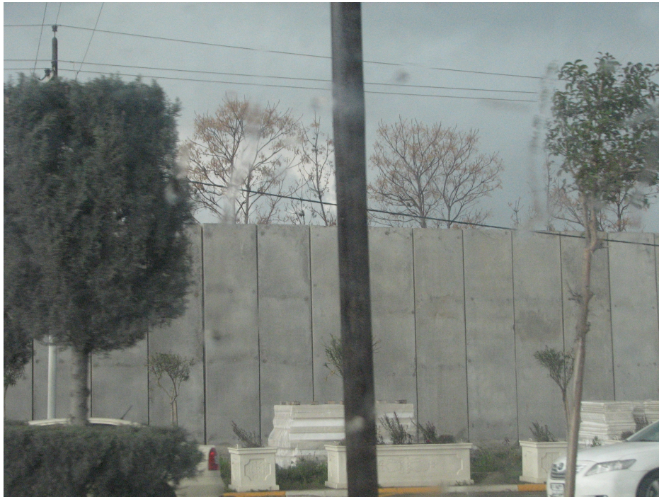
Figure 11: T-walls eclipse a shorter brick wall around a police headquarters in Erbil, photo by Kali Rubaii
