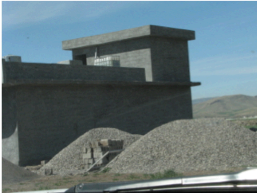
Figure 22: The Jowad's "house" near completion in 2015, photo by Kali Rubaii
