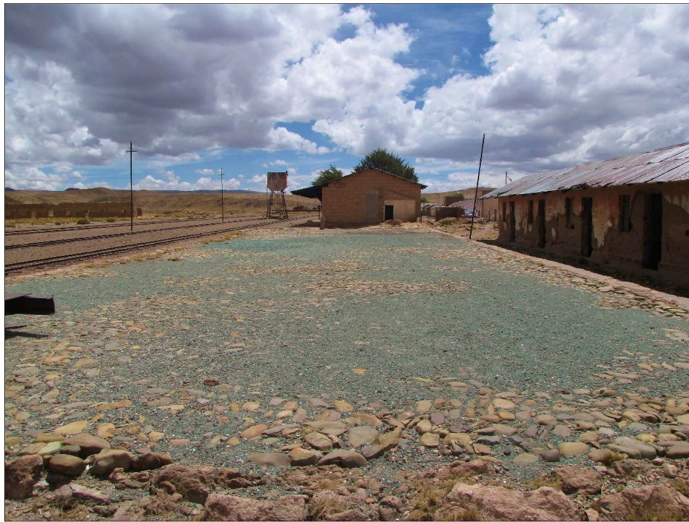
Figure 3.4: Loading platform at the Calacoto Station covered with mineral (Photographed by author in 2012).
