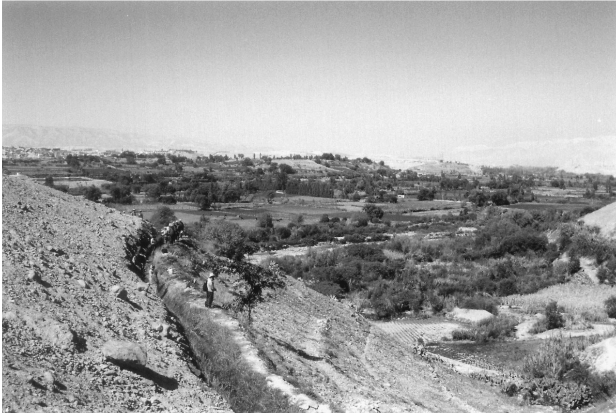
Figure 16.2. Modern agrarian immigrant community constructing canal, Moquegua, 2005.
