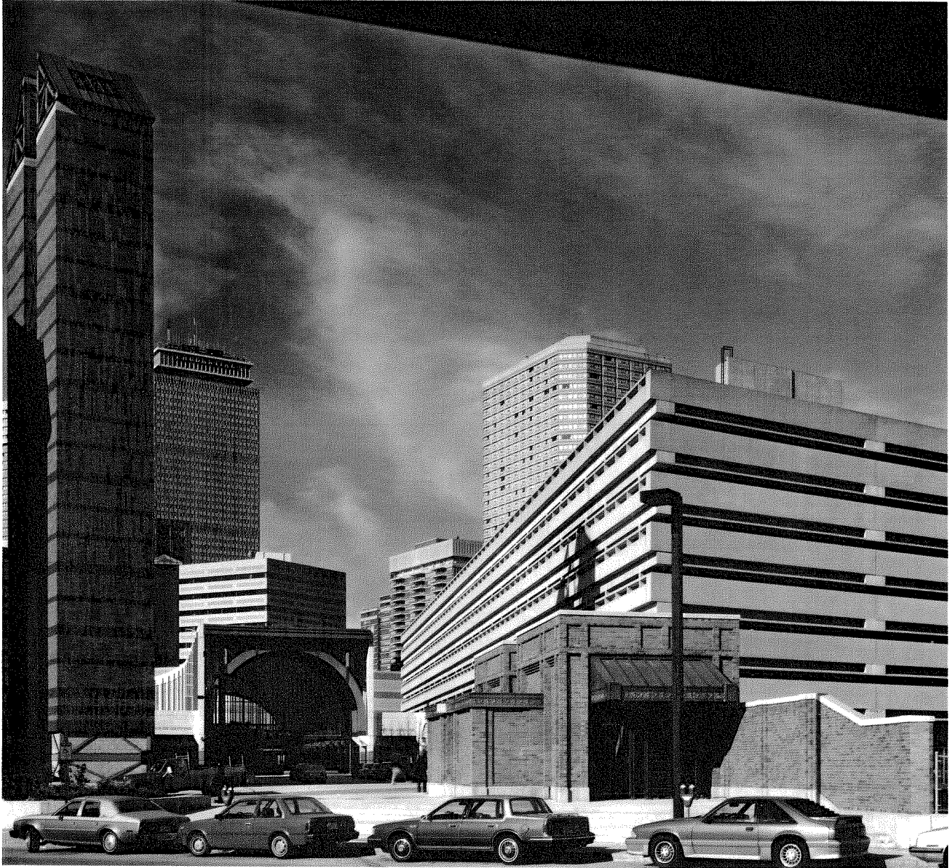
I Back Bay/South End station in Boston. The venting towers, the main hall, and the brick exitway kiosk viewed from Columbus Avenue looking west. Photograph by Steve Rosenthal
