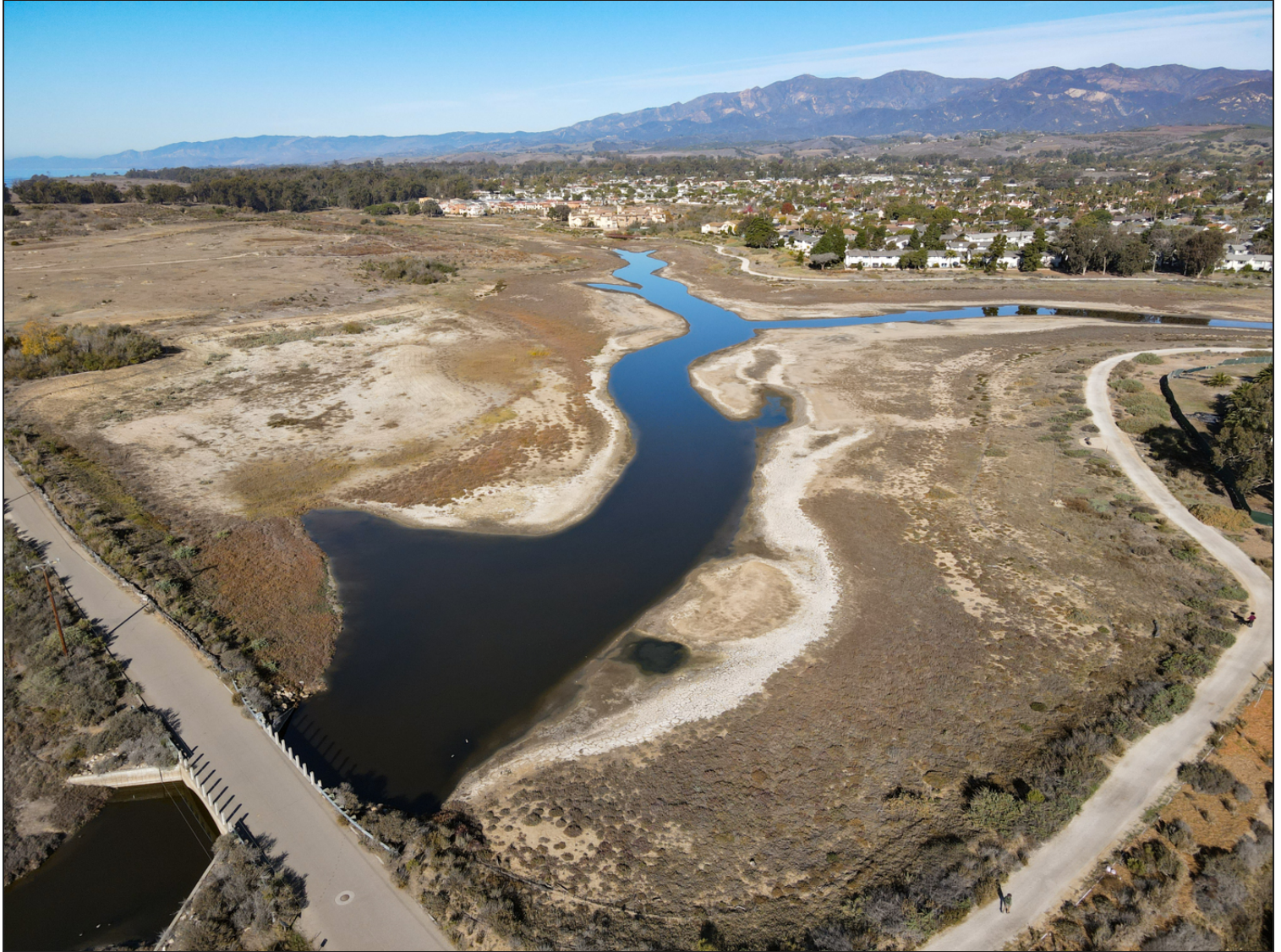
NCOS aerial photo taken on 11/18/22.
