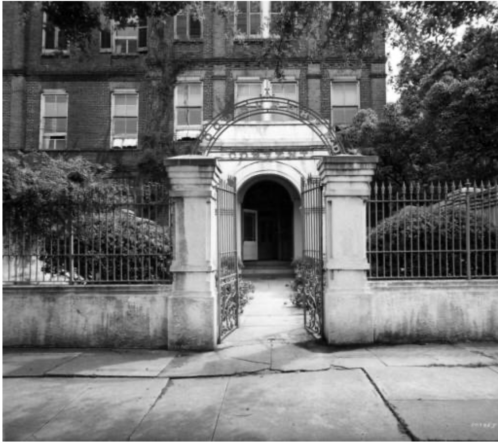
Figure 0.2: Charles L. Franck, House of the Good Shepherd, Entrance Gate , Charles L. Franck Studio Collection, The Historic New Orleans Collection, 1956. 1979.325.2262.
