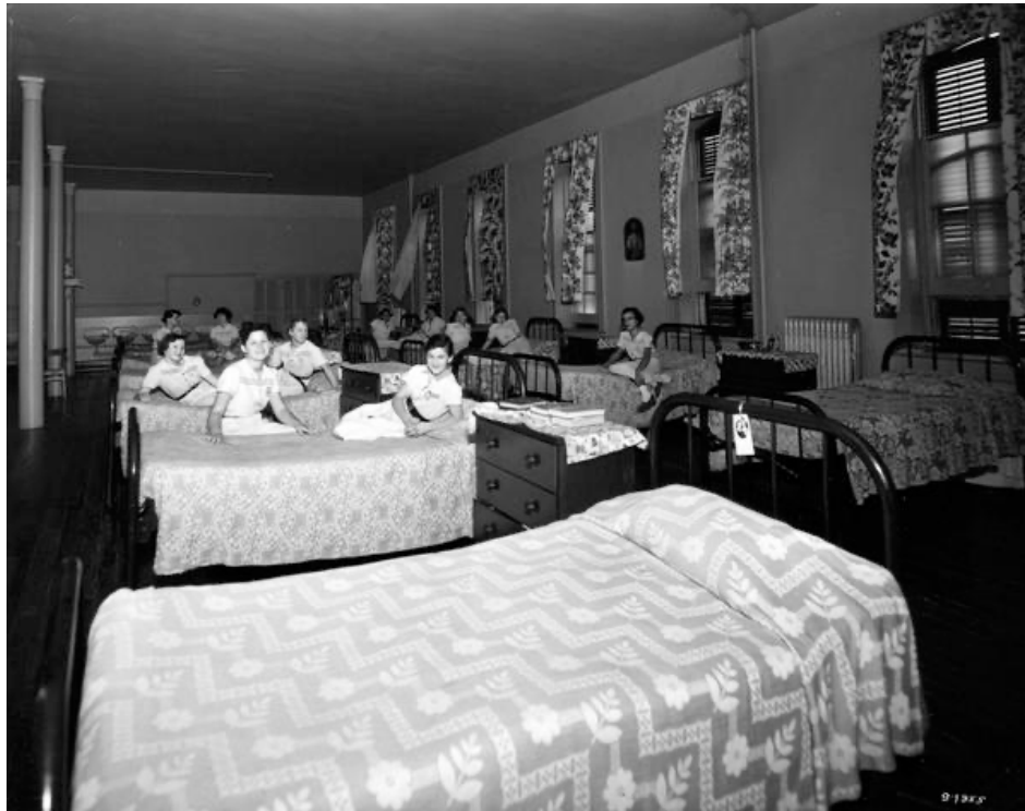
Figure 3.15: Charles L. Franck, House of the Good Shepherd, Dormitory . Charles L. Franck Studio Collection, The Historic New Orleans Collection, 1956. 1979.325.2270.
