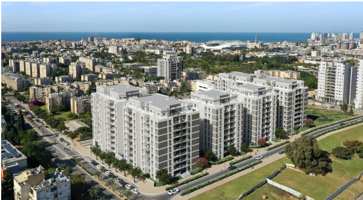
Figure 53: A render of 'The Gadna' project in Mevohot Jaffa. Source: The Gadna Tel Aviv. Renten.
