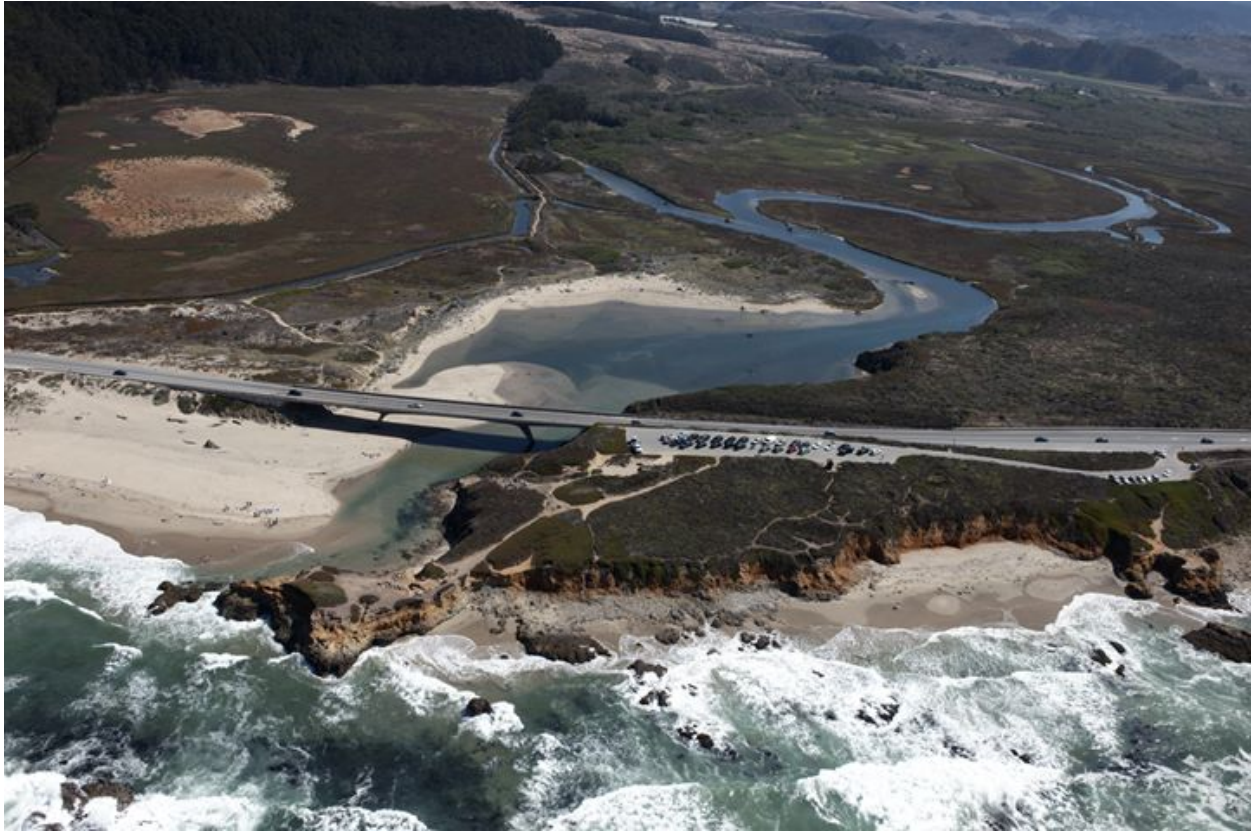
Figure 2.1: Photograph of the Pescadero Beach and Natural Marsh Preserve. The Highway 1 bridge crosses the shallow inlet of the estuary. Butano Creek arrives to the confluence of two creeks from the right of the image through wetlands. Pescadero Creek is more wooded and channelized. Photograph taken Sept. 25, 2010. In 2010 the inlet closed in October. Copyright ©2002-2013 Kenneth & Gabrielle Adelman, California Coastal Records Project, www.californiacoastline.org .
