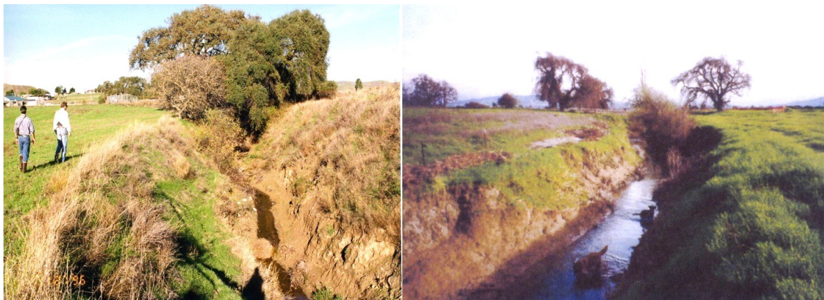
Figure 3. Pre-project photos showing incised conditions
