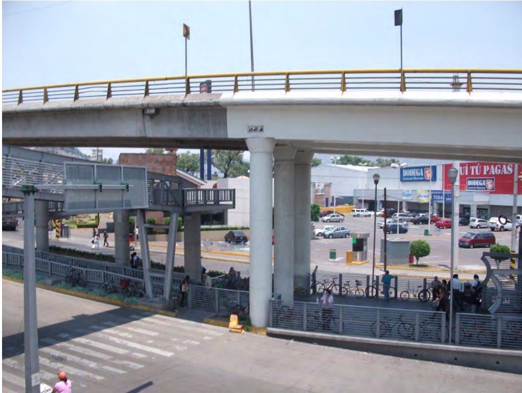
Figure 2.20 Pedestrian bridge crossing at Tenayuca Metrobus station (2012)
