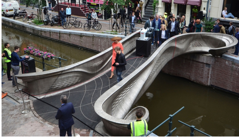
Figure 4: MX3D Bridge in Amsterdam [15].
