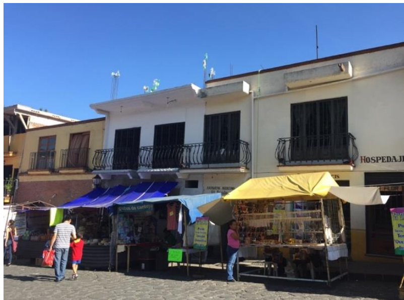
Figure 45. Decorative faux balconies installed along frontage.
