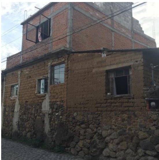
Figure 43. Adobe construction with brick second story added.
