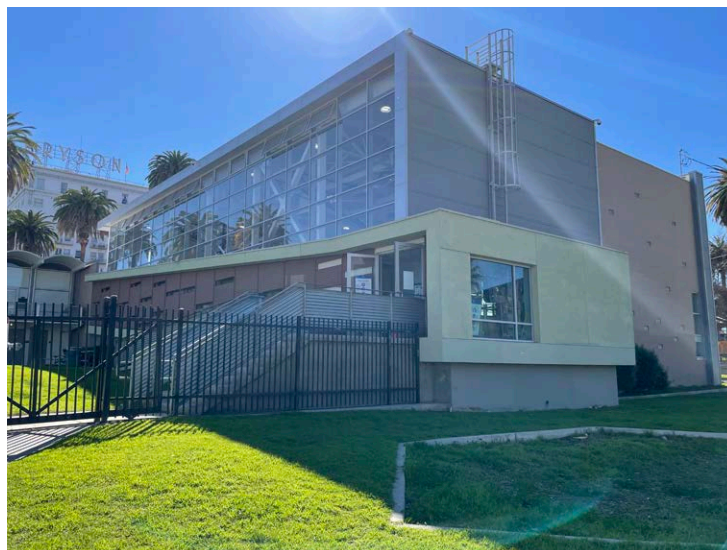
The Lafayette Multipurpose Community Center. During this research study’s observation period, the Center was not open to the public.
