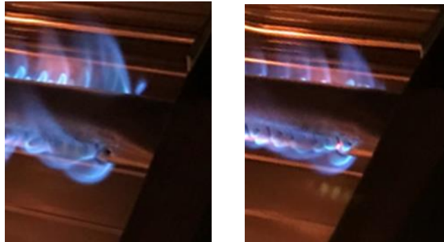
Figure 43: Over-heated oven burner part at 20% hydrogen addition
