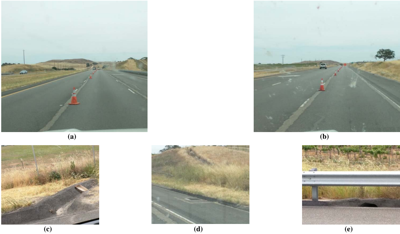
Figure 4.55: Site and drainage conditions at San Luis Obispo 46 in May 2016.
