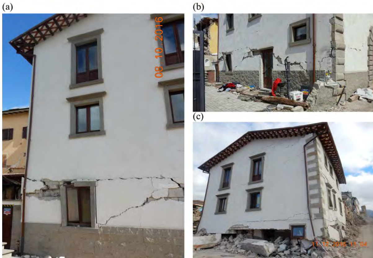
479 Figure 18. Residential masonry residential building after the 24 August earthquake (a, b) and (c) after 480 the entire sequence. Shear failure of the ground floor bearing wall leads to soft story collapse at the 481 end of the third event.
