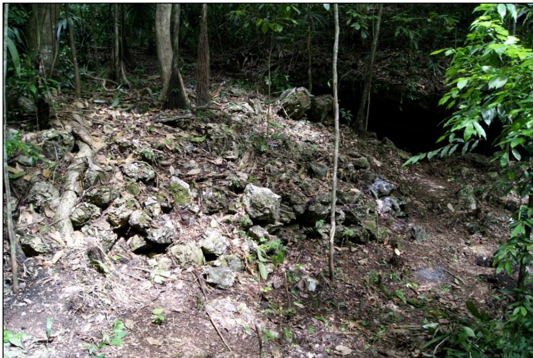
Figure 6. Showing the terrace wall to the left (East) of the cave entrance.
