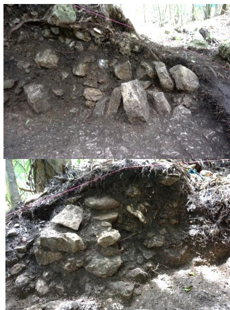
Figure 68. The front of this structure has visibly collapse outwards at the southwest corner. The northern edge of the unit shows better preservation with vertically stacked stones still visible in profile.
