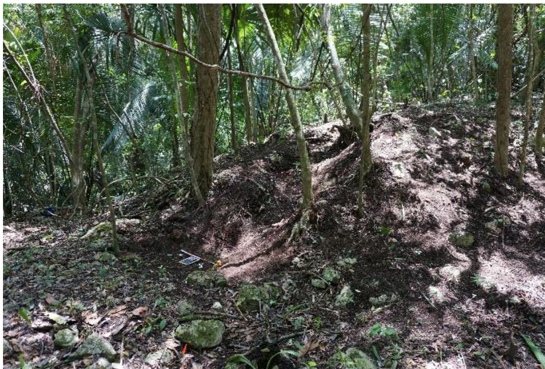
Figure 66. Unit 2 was placed in a visible looters trench in order to provide quick access to assess the construction technique of this structure.
