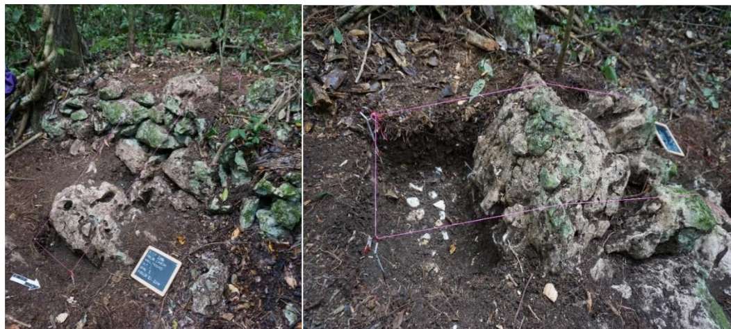
Figure 128. Figure 95. The construction of the terrace wall showing the fill on top of the terrace.
