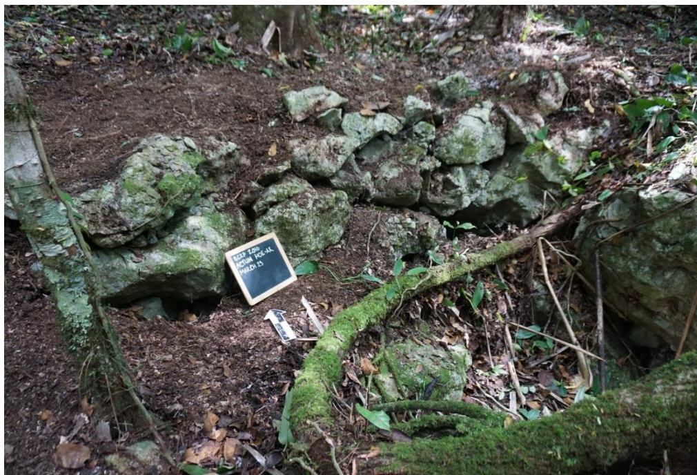
Figure 134. The terrace wall next to the cave entrance where Unit 1 was placed.
