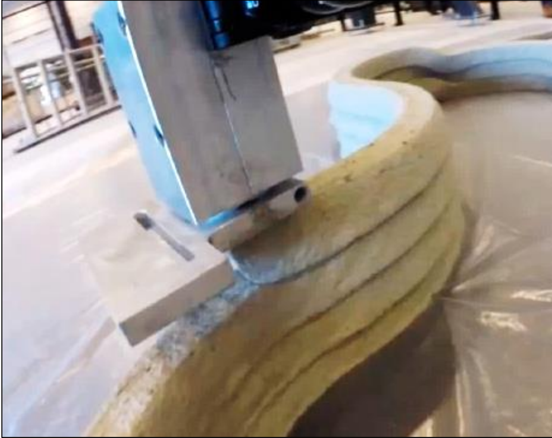
Figure 2.1: 3D concrete printer in operation. No-slump concrete leaves the nozzle as a relatively stiff continuous filament. [23]
