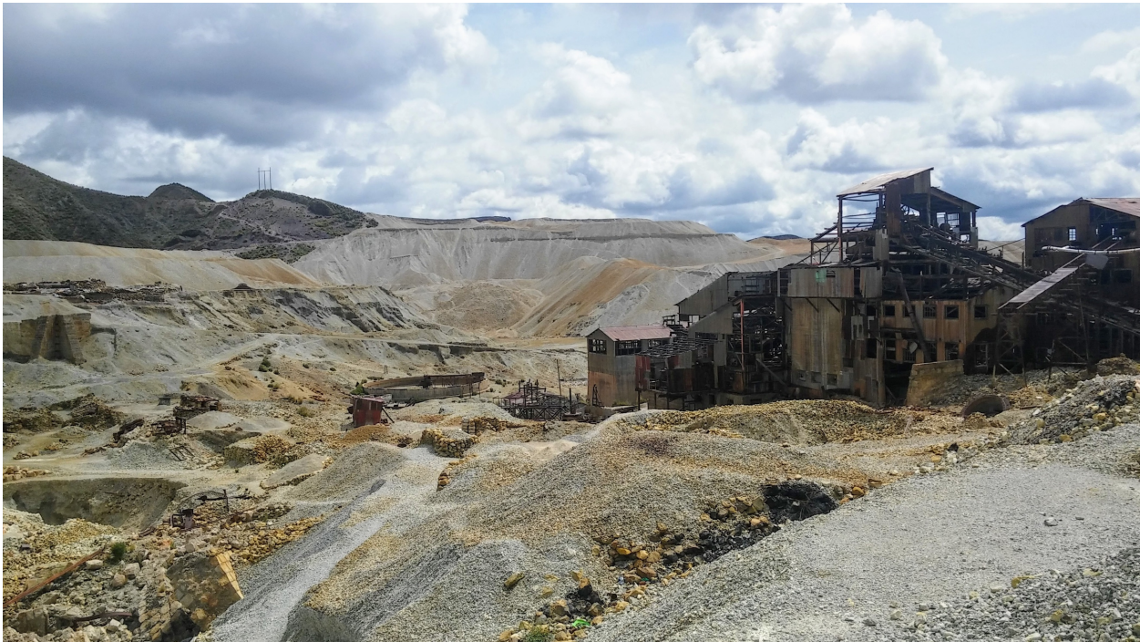
Figure 22: Sink & Float Plant amid desmontes , Llagagua. March 1, 2016.
