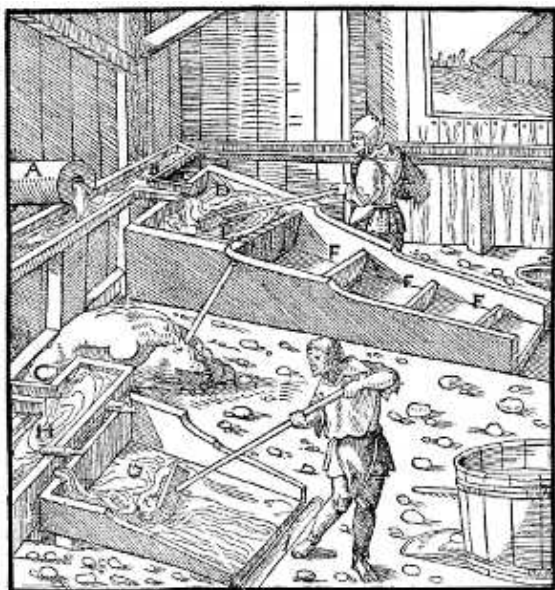
Figure 25 (left): Buddles as featured in De Re Metallica (Agricola, 1556: 302).
