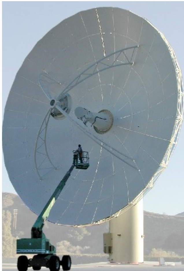
Fig. 6-21. Reflector antenna constructed with large pseudo-rectangular subpanels, from http://www2.1-3com.com/datron/ .
