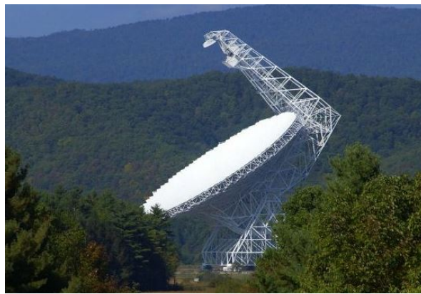
Fig. 1-1. The Green Banks 110 m radio telescope is the largest fully steerable antenna. (Photo from www.gb.nrao.edu .)
