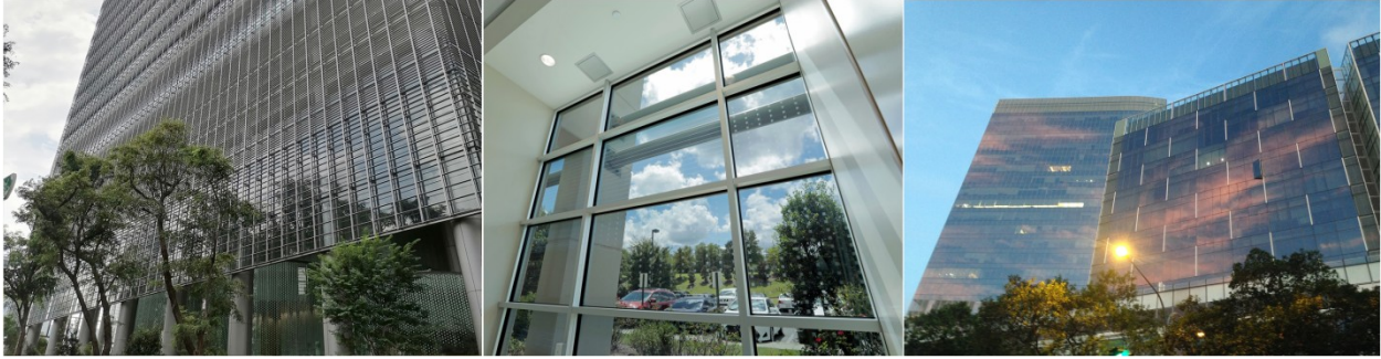
Figure 8 Three different facades showing: solid shading solutions created by external louvres with low view clarity and a Threat Factor of 5; bird-safety glazing installed on an airport façade 144 with continuous frit patterns and a Threat Factor of approximately 25; and unobstructed fully glazed façade with high view clarity and a Threat Factor of 100
