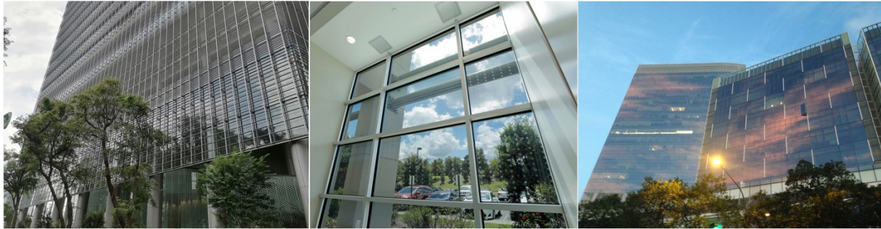
Figure 8 Three different facades showing: solid shading solutions created by external louvres with low view clarity and a Threat Factor of 5; bird-safety glazing installed on an airport façade 144 with continuous frit patterns and a Threat Factor of approximately 25; and unobstructed fully glazed façade with high view clarity and a Threat Factor of 100
