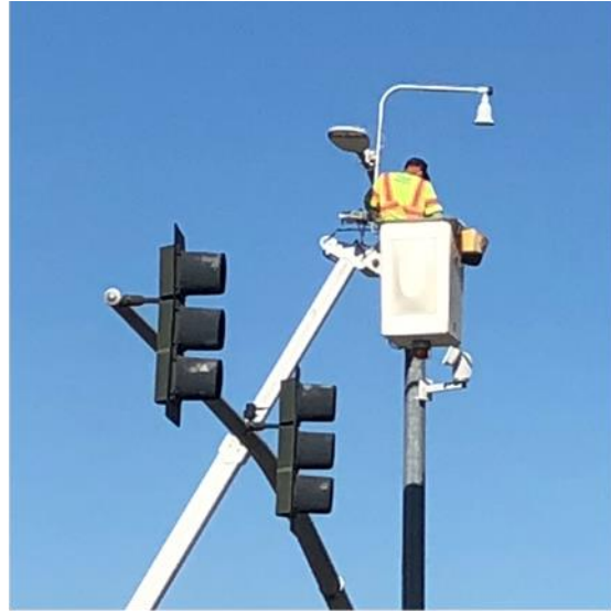
(b) Installing Camera on Street Lamp Post
