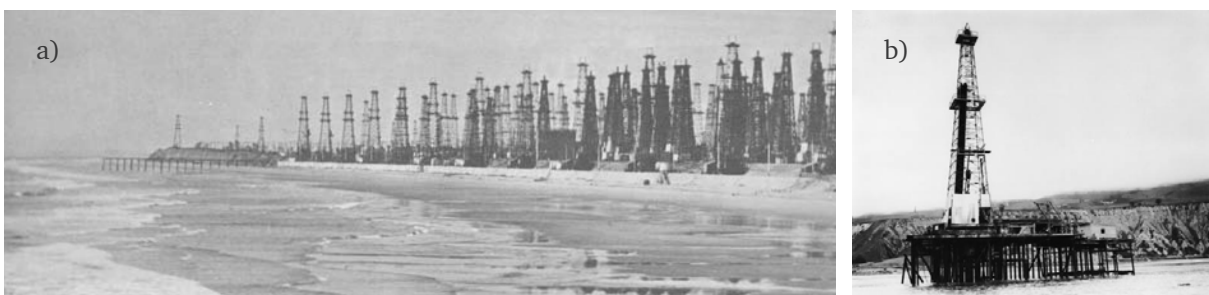
Figure 2.3-3. (a) Huntington Beach (1932) - first directional drilling from onshore under the ocean. (Wentworth, 1998); (b) Steel Island (1932) – first offshore platform. (Love, 2003).
