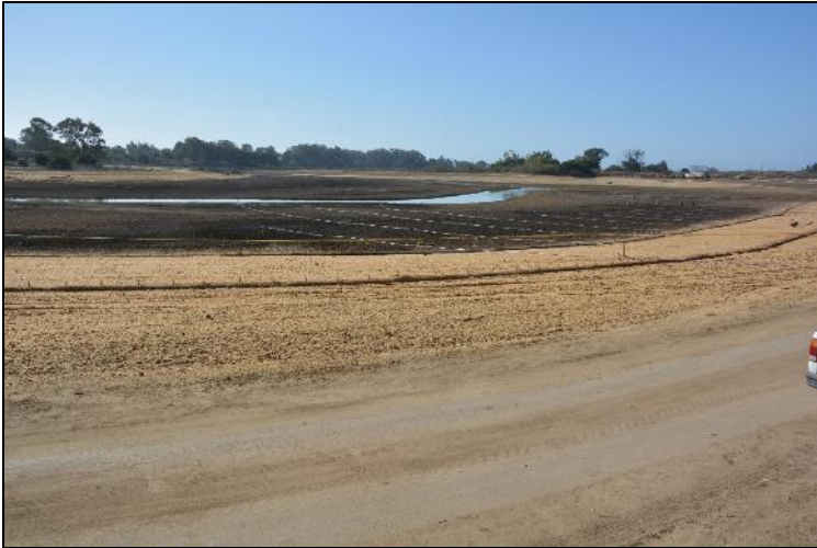
Baseline (post-grading) - October 2017
