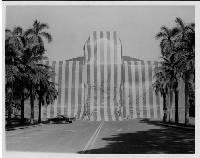
Figure 4 Termite tenting during the restoration by the Friends, circa 1960s. Courtesy Hawaii State Archives, Photograph Collection.
