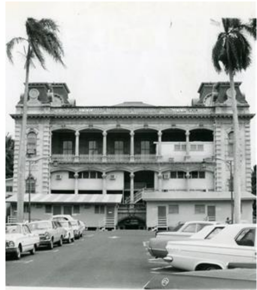
Figure 2 Additional temporary extensions were added on the rear lanais (porches) of the Palace. Courtesy 'Iolani Palace Facebook Page, January 26, 2019, Accessed February 2, 2020.
