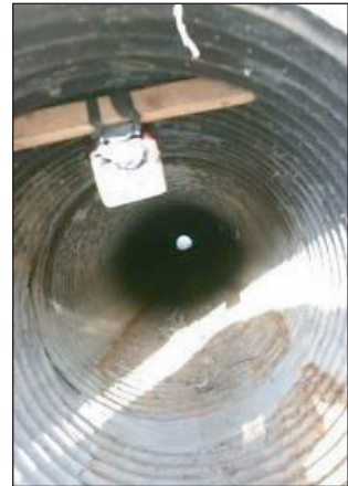
Figure 5. Installed camera in circular culvert
