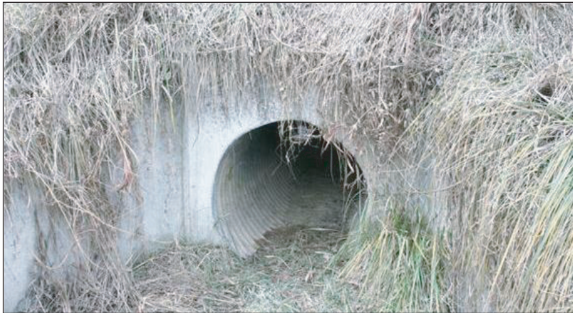
Figure 4. Circular culvert (waved steel pipe)
