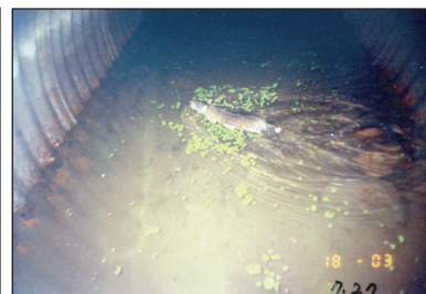
Figure 7. Inundated circular culvert.
