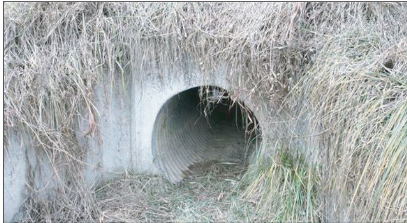
Figure 4. Circular culvert (waved steel pipe)
