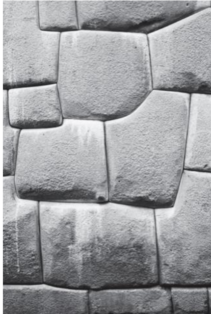
Figure 1.14. Inka wall of nibbled, high-status polygonal masonry, Compound of Inka Roqa (Archbishop's Palace), Cusco, Peru. Image from: Dean, Culture of Stone , 116.
