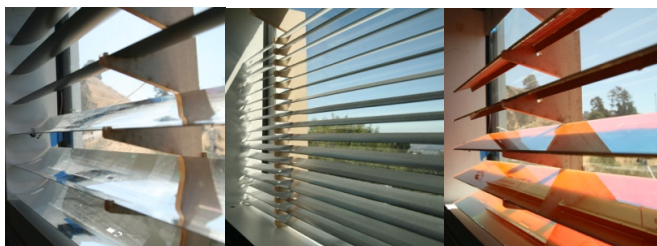
Figure 3. Close-up view from the interior of (left) curved specular slats, (center) curved prismatic slats (right) and flat specular slats.
