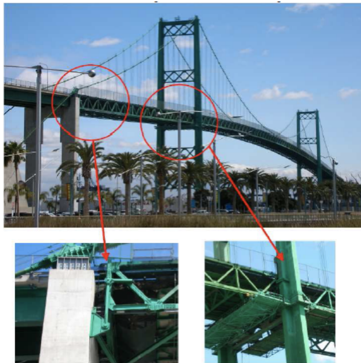
Figure 7. Bridge Dampers detail on real structure
