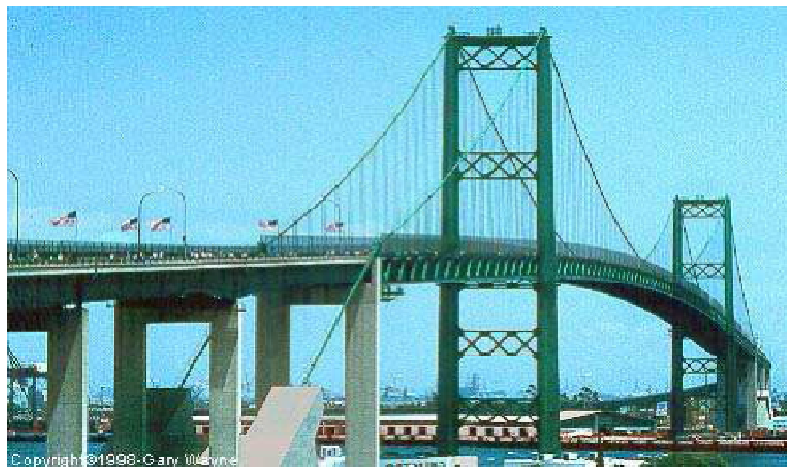
Figure 1. The Vincent Thomas bridge
