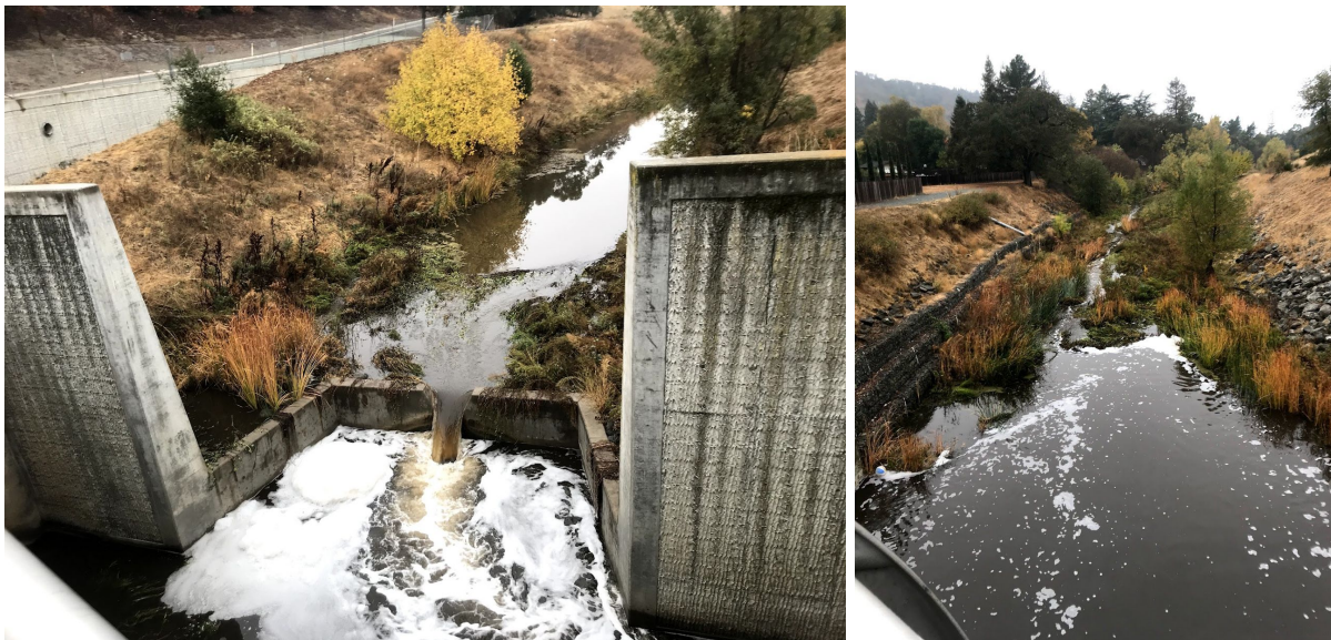
Figure 9: San Ramon Creek at Livorna Rd. (a) Left: Concrete drop structure. (b) Right: Downstream view.
