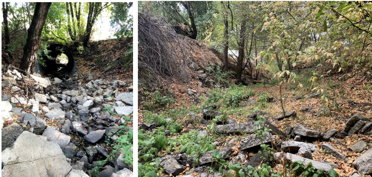
Figure 13: (a) Facing downstream, corrugated metal pipe culvert. (b) Facing upstream with riprap.
