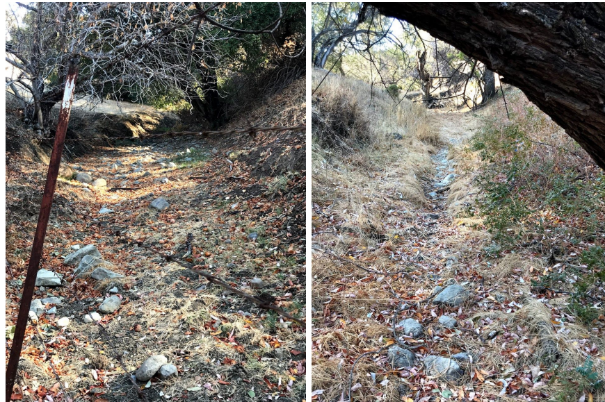
Figure 17: (a) Left: Facing upstream. Earthen trapezoidal shape. Bound by fence. (b) Right: Facing downstream. Channel becomes narrow and shallow.
