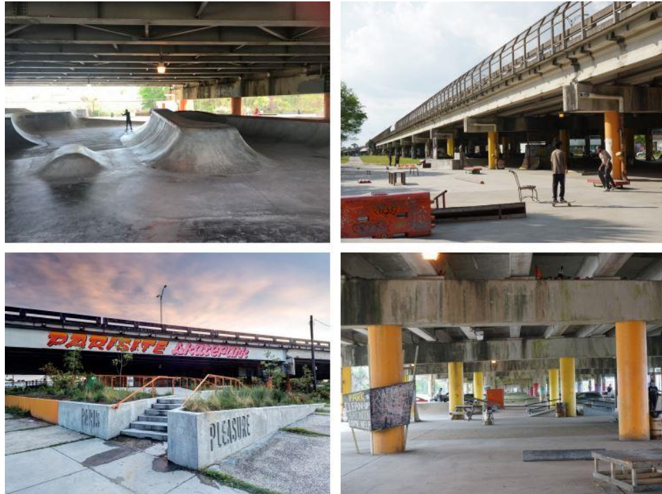
Figure 2. The entry and stormwater garden, the "peanut pool," an area for street-style skating, and bays offering ramps for transitional skating. Photos by Michael Wong (Wener, 2020)
