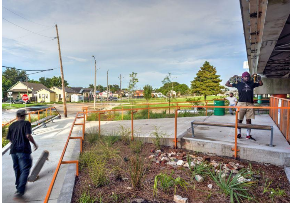
Figure 3. Bounded bays and integrated stormwater garden (Wener, 2020)
