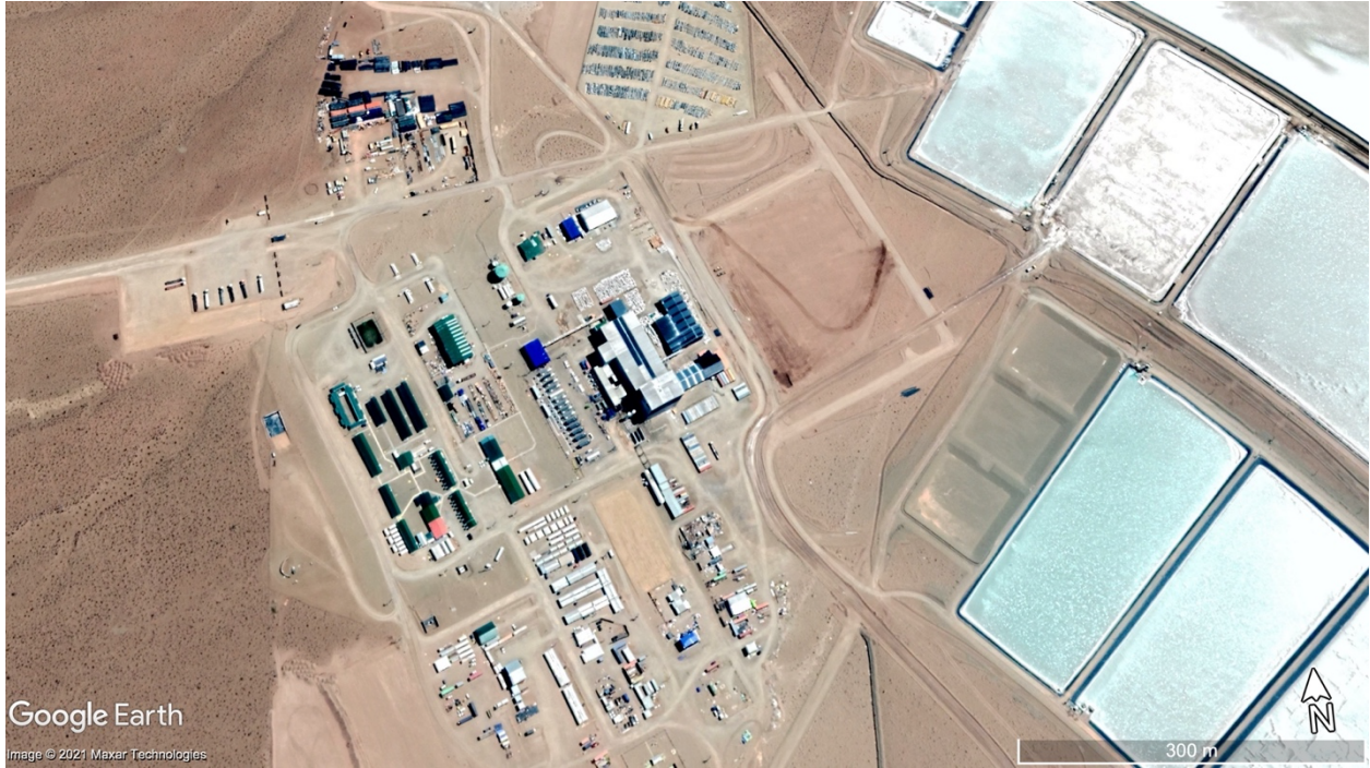
Figure 10. This image is from Google Earth Pro’s historical time series data which shows the Sales de Jujuy operations site in 2020. The image was captured at an altitude of 5,000 m.
