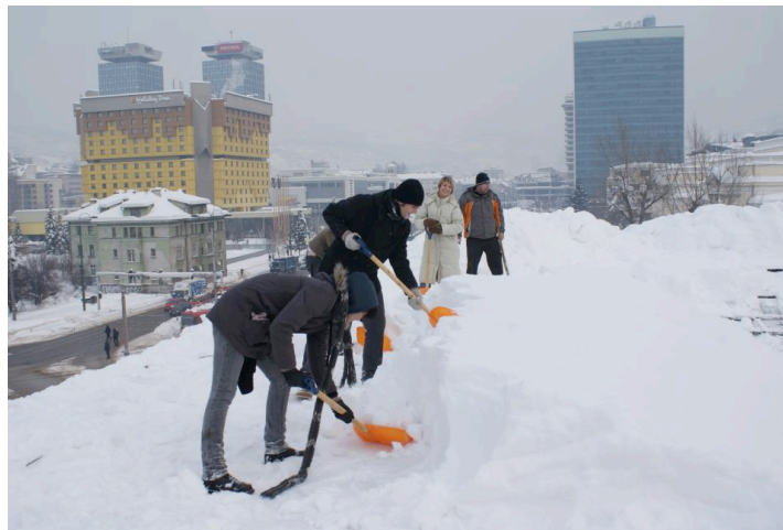
Figure 39: Members of Citizen Action remove record snowfall from the roof of the Historical museum, to prevent its collapse. Photo courtesy of Elma Hašimbegović
