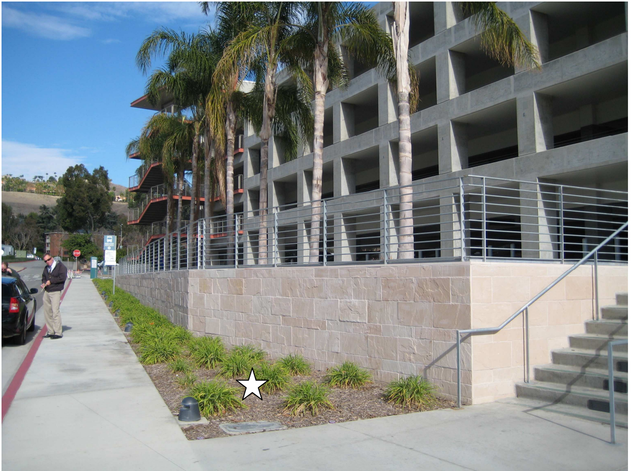
Figure D.2 Location of the Bus Stop at the Parking Structure
