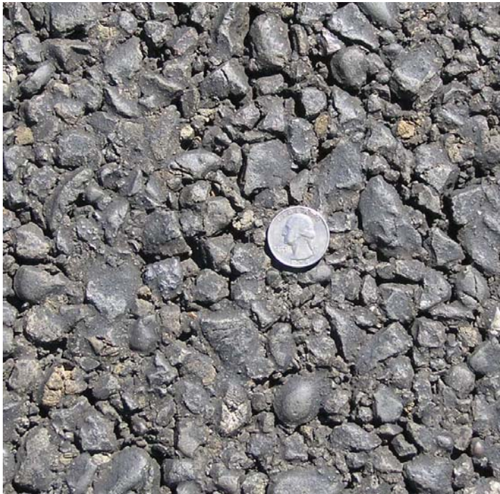
Figure 14: Rubberized open-graded asphalt concrete F-mix (RAC-O F-mix).
