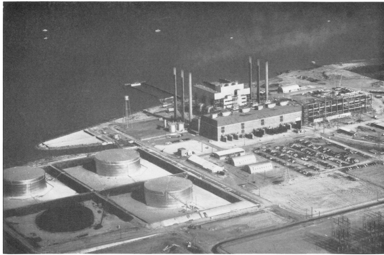
FIGURE 2. Aerial photograph of the Contra Costa Steam Plant, showing construction in progress for Units 4 and 5. Cooling water intake structure in the river is north of the boiler building for Units 1, 2 and 3. Cooling water discharge is shown immediately above fuel oil tanks. Photograph by P. G. & E. News Bureau, November, 1951.
