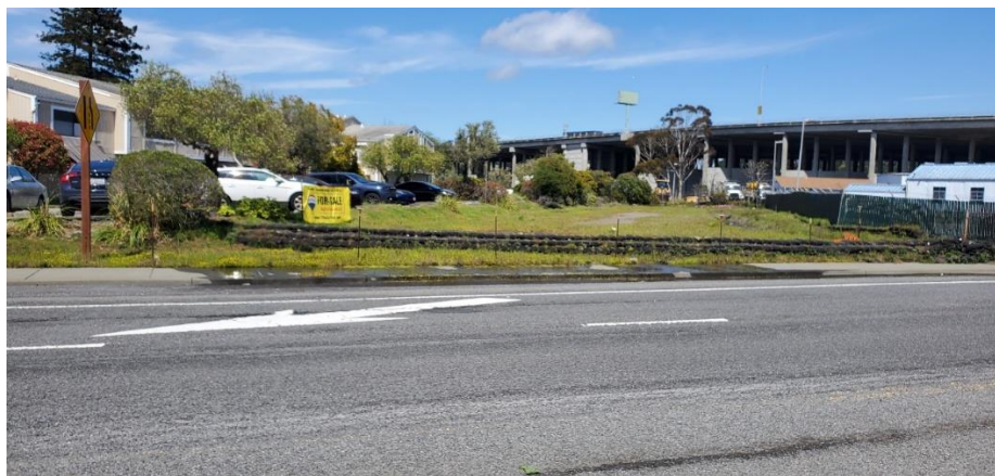
Figure 3.11: Manzanita emerging groundwater pouring over sidewalk April 15, 2024. The location is directly above a preferential flow pathway (sewer utility trench).
